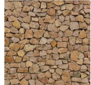
Loose Stone Wall
