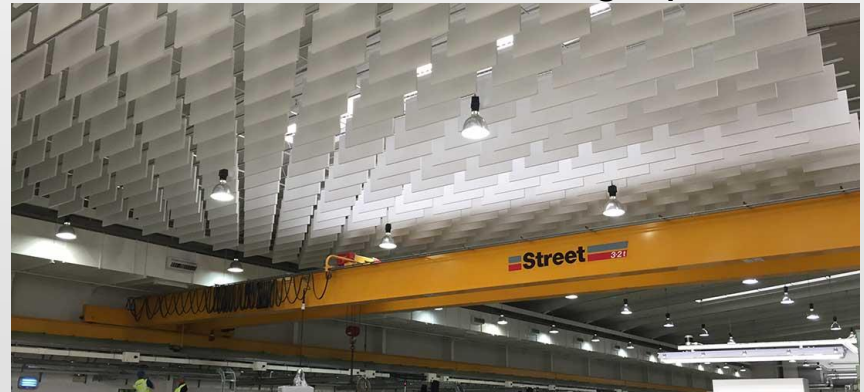
Baffles in Manufacturing Space
