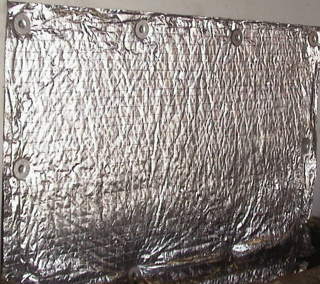
Curtain wall insulation fastened to steel angle Project R Value drive insulation thickness (2-6" Typical)
