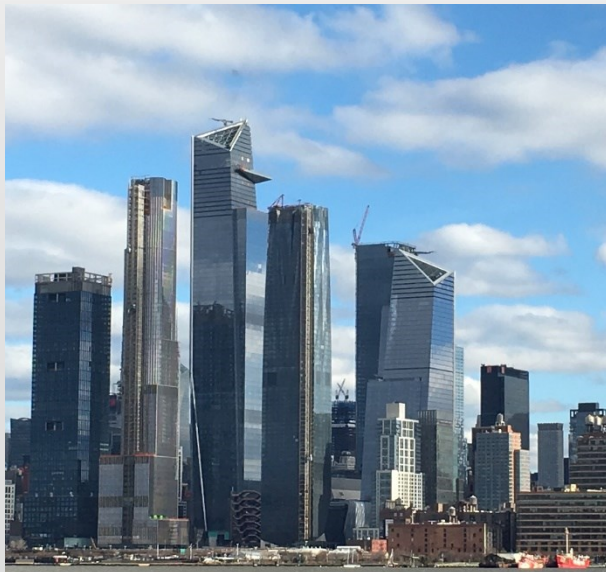
NY, Hudson Yard Tower C
