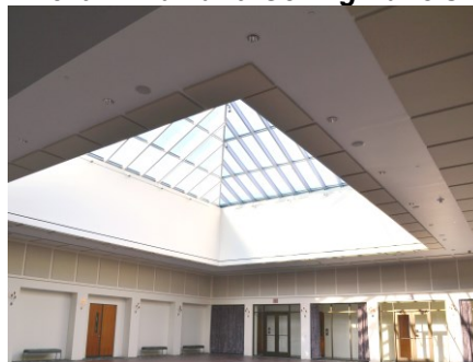
Atrium Wall and Ceiling Panels
