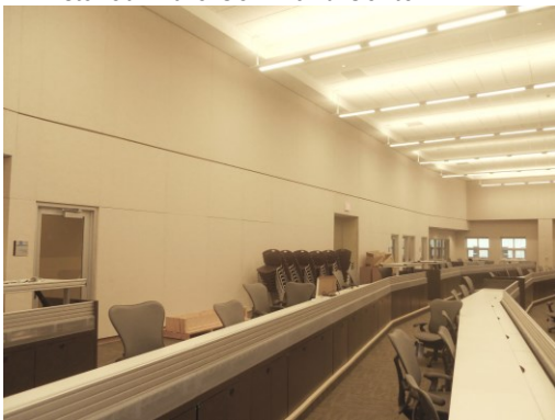
Absorption Plus Impact Wall Panels Installed in the Command Center.
