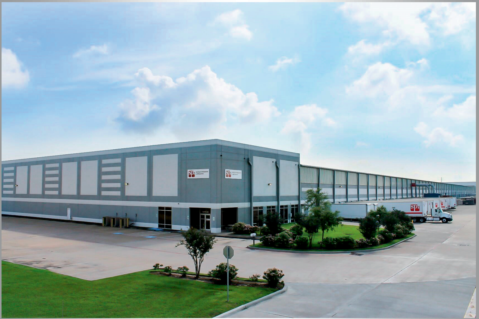
SPI Distribution Center and Fabrication Facility, La Porte, TX - USA
