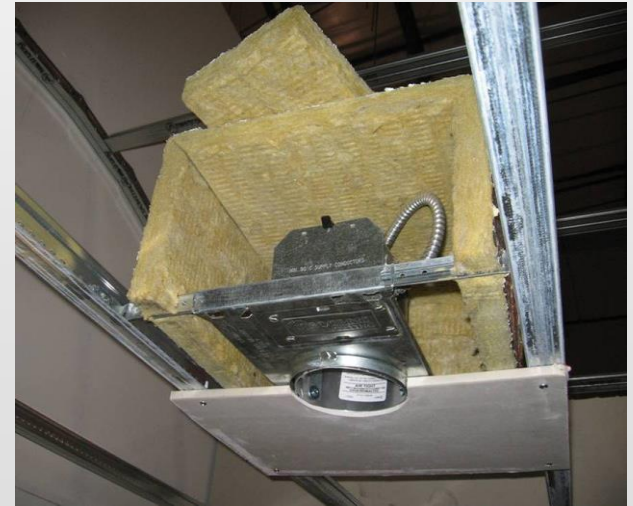
SafeLite Enhanced Fixture Insulation
