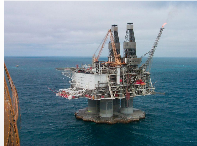
Hebron Platform - 1600 SafeLite installed on lights and speakers
