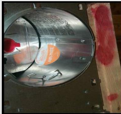
Per CODE, “Air-Tite” but NO Insulation Value
