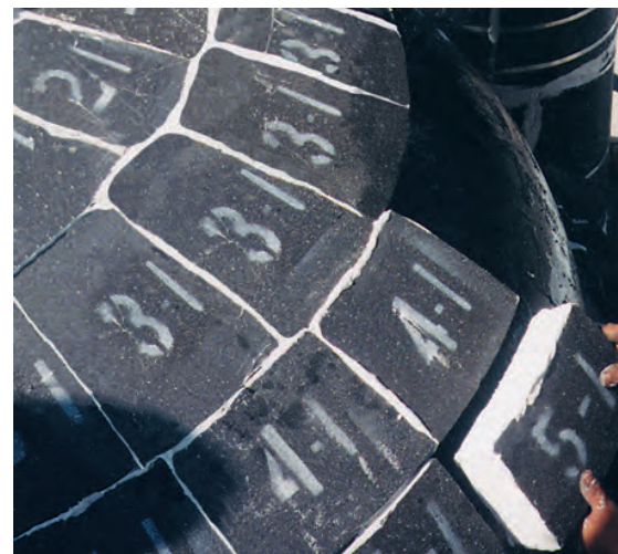
Pamrod HATS were installed while this cryogenic tank was in operation.
