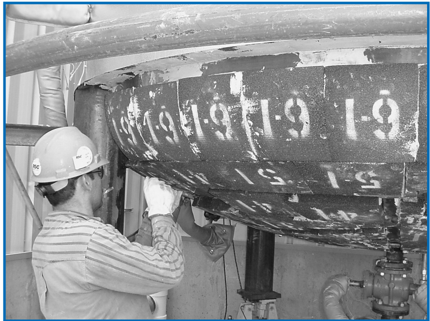
Installed in concentric circles, Pamrod HATS segments are numbered for easy installation.
